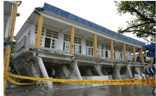
In-situ pushover test to verify the proposed technology for seismic evaluation and retrofit of school buildings
